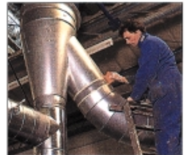
SEAL SPLIT DUCTING
